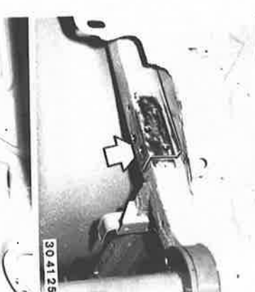
Uncover mating surfaces of left and right side members. Drill off welding spots. Lift out trunk floor plate complete with side members.
