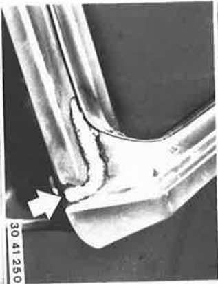
Braze and grind down joint between side panel and tail panel.
