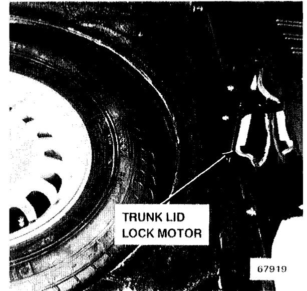
Figure 5 - Middle Rear of Trunk
